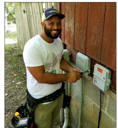
Jonathan Noel, in-home fiber installation tech.
